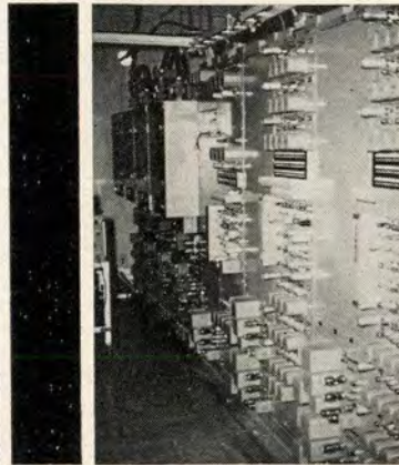
Fig 4, left, tropo site with transmission equipment. Tubes and checkpoints are accessible from exterior, eliminating working "in the blind."
