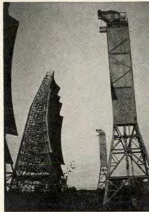
Fig 3, right, the Mark 85 tropospheric scatter antenna reaches 118 feet into the air and requires maintenance in all kinds of weather.
